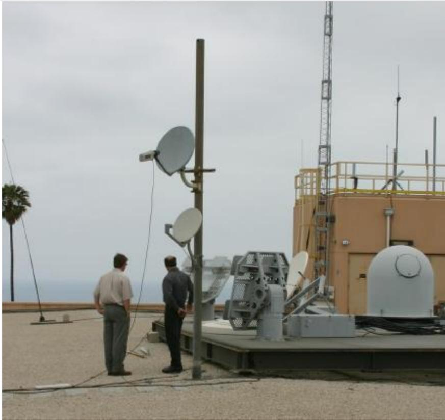
The antennas will have a mounting platform compatible with that pole. The link to Mt. Soledad will use a similar setup, likely with a 4' antenna. We will need to either utilize indoor space for the radios, or mount a weather-resistant box onto the roof, possibly the steel structure. All equipment is powered by 110V AC.
