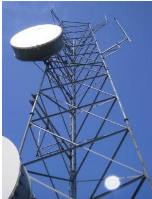
The FCC imposed limit for the license-exempt 5.8GHz band is 53dBm EIRP. The antenna has an about 40dBi gain, and the radio can be software-configured to match the 53dBm limit, taking antenna gain and connector/cable loss estimates into account.
